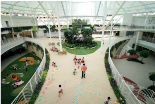
Figure 7 Yishun Community Hospital. © CIAP Architects.
