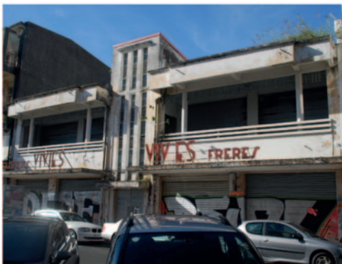
■ 7 - Garage Vivies, quai Lefebvre, 1949
